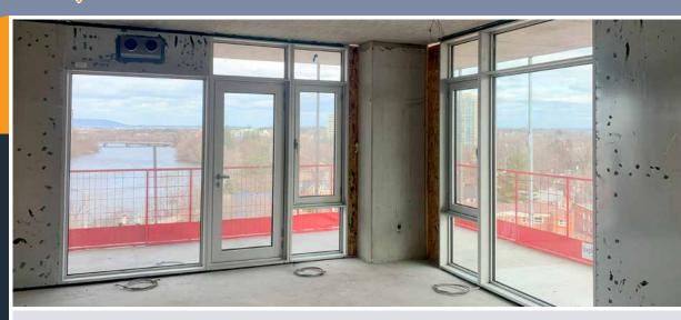
In our latest update, we celebrated topping off the 22-storey first tower with the installation of its final structural roof plate, marking a significant milestone in our progress. Concurrently, the installation of precast elements and punched windows added to the tower's striking appearance, while ongoing work on demising walls ensured the interior spaces took shape.
